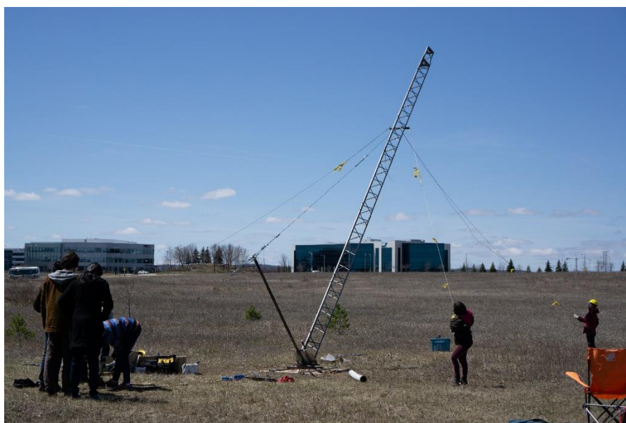
Figure 13. Launch tower raising. This photo depicts the launch tower as it is being raised. The gin pole can be seen at the base of the tower.
